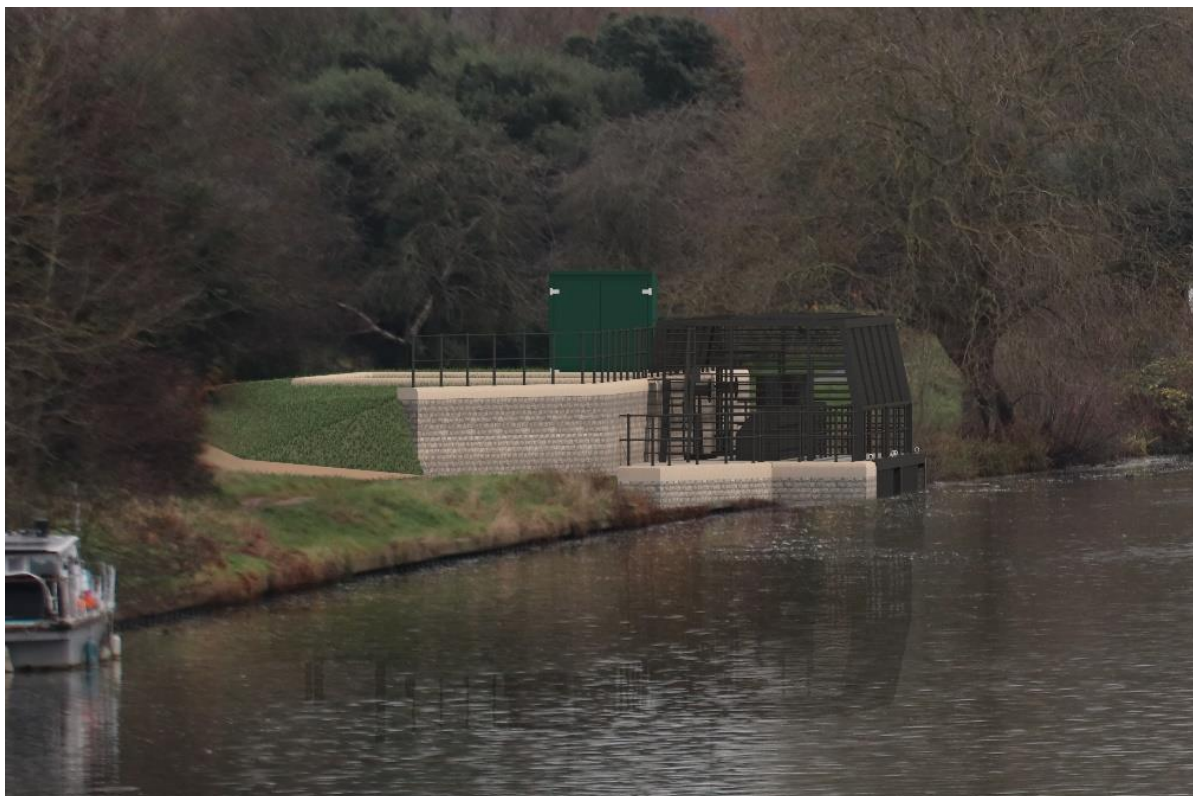
Figure 2.10 An indicative image of an intake structure upstream of Teddington Weir
