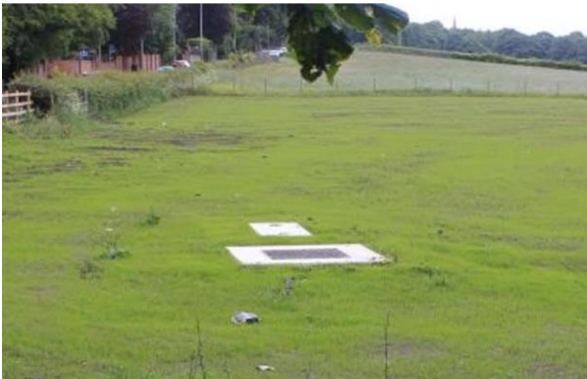
Figure 2.11 Typical shaft access hatch after completion
